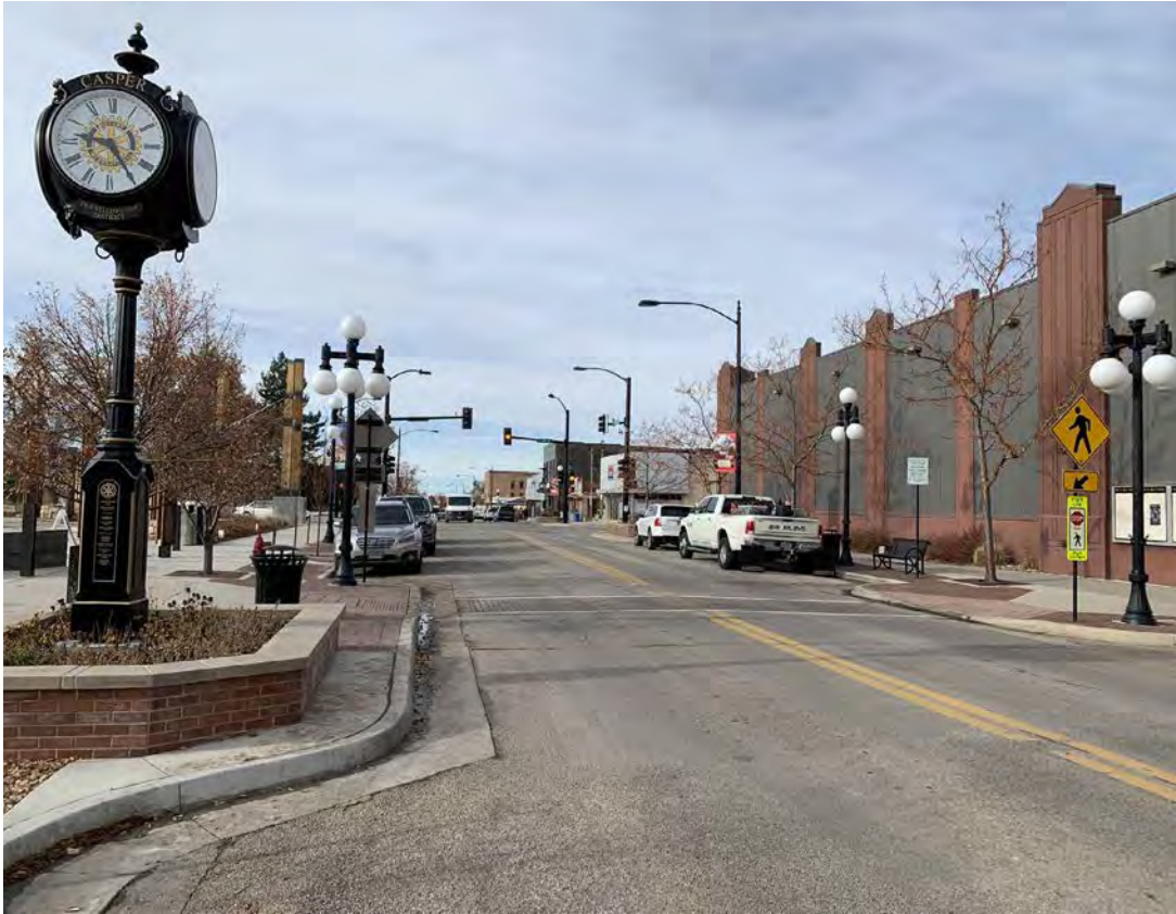
Midblock curb extensions at David Street Station
