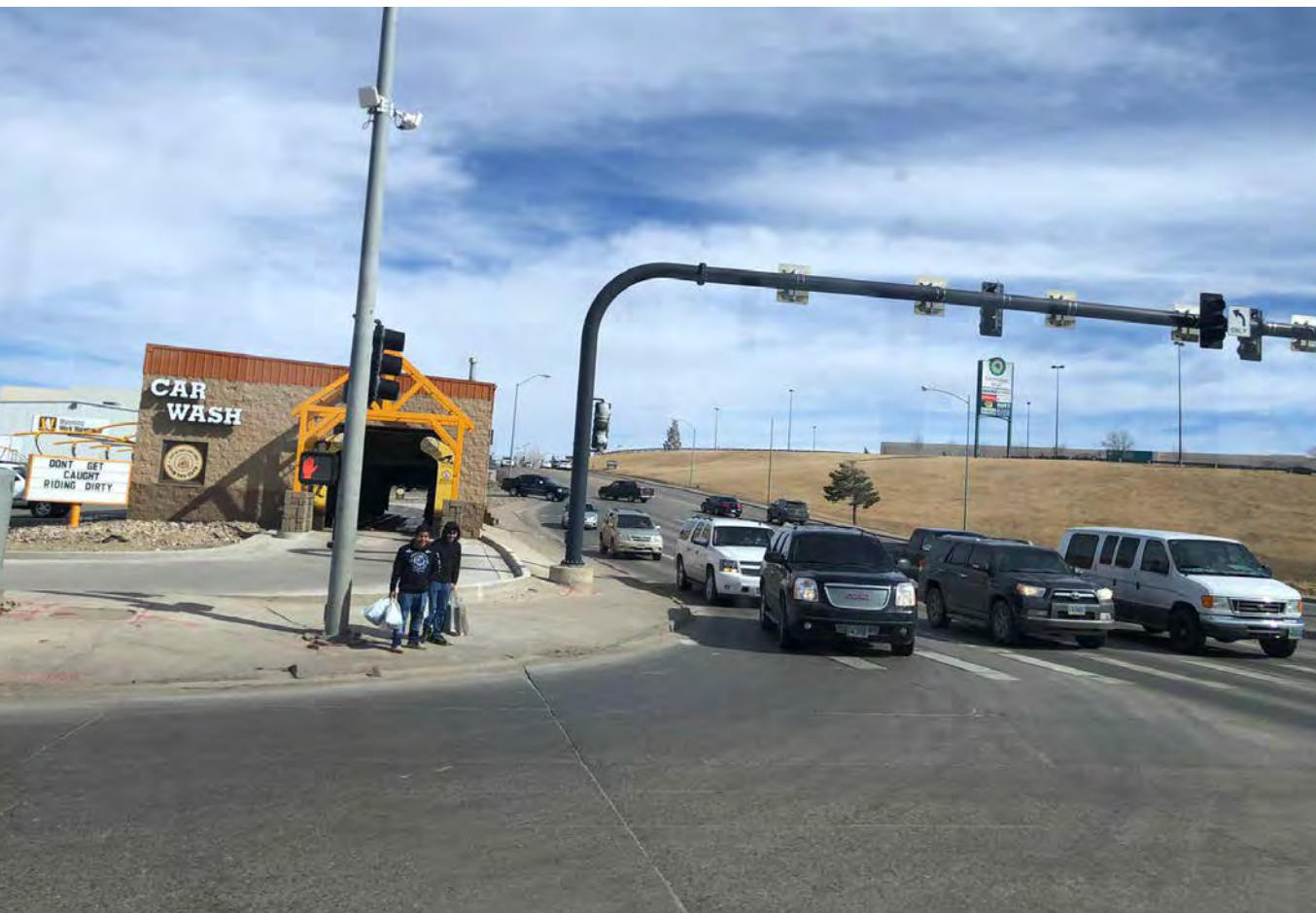
Some larger intersections, such as E. Second St and Wyoming Blvd shown here, have long crossing distances with a lack of pedestrian safety counter measures such as curb extensions, high visibility crosswalks, and refuge islands.
